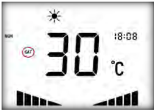
Supply Air Temperature
