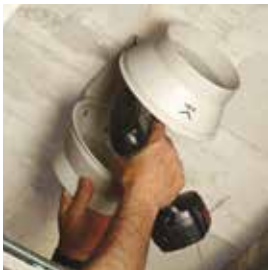
Fix the support bracket.
