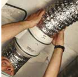
Connect the ducts.
